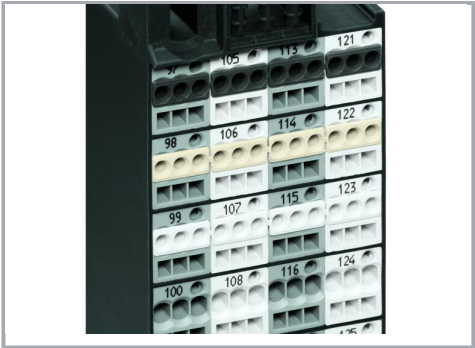
Insulation stop is in place.
